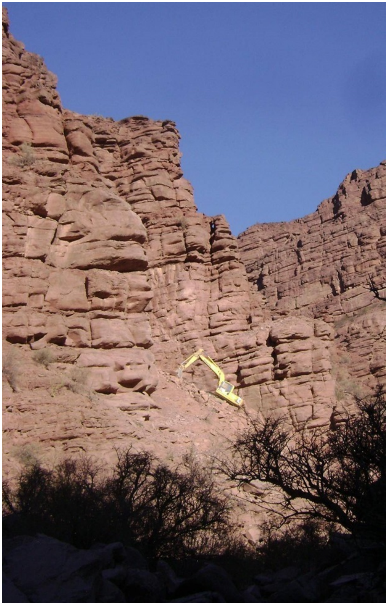
One of the few interventions on the red sandstone walls of the Agua de la Peña Canyon. Tunnel roads were located 150-200m away from the walls, parallel to the canyon course.
